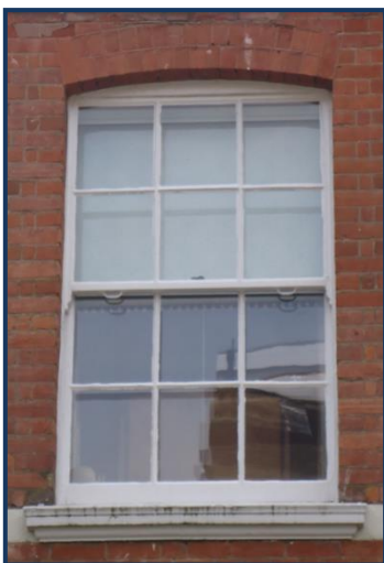
Traditionally formed timber sliding sash windows
