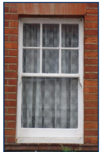
Traditionally formed timber sliding sash windows
