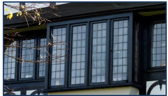
Left: Top hung hinged casements with centrally located fixed lights Right: Side hung hinged casements with centrally located fixed lights
