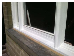
A traditional repair in situ
